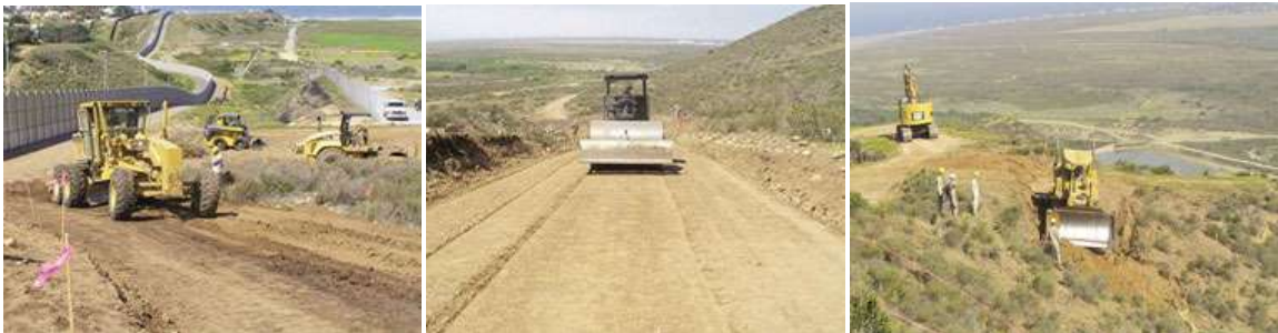
The steep slopes on the west side of Bunker Hill presented a significant challenge as the slump of the concrete varied from three to five.
