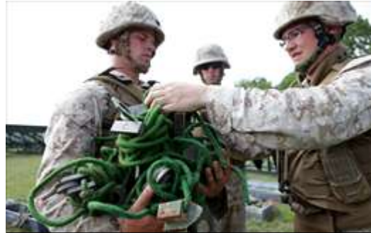
Cpl Colin Smith, a combat engineer with Bridge Co. C, from Memphis, hands out pieces of equipment to build a medium girder bridge during a training exercise here, June 11. The process of putting together an MGB can take upwards of 30 Marines and nearly a day to assemble properly. (Photo by Cpl John M. McCall)
