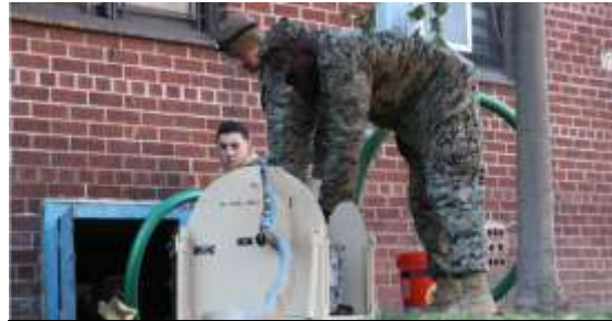
Marines with 8th ESB, 2nd MLG get ready to start a gas-powered pump to remove water from a flooded basement while conducting humanitarian operations in Far Rockaway, N.Y., Nov. 4. Approximately 86 Marines from the unit were deployed to New York to help pump water from flooded areas of the state. (Photo by LCpl Scott W. Whiting)
