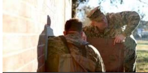
Sgt Justin Armstrong, a Marine with 8th ESB, 2nd MLG, and GySgt Justin Gober, a Marine with 8th ESB, 2nd MLG, examine the depth of a basement in order to pump water out into the street while conducting humanitarian operations in Far Rockaway, N.Y., Nov. 4. Approximately 86 Marines with 8th ESB, 2nd MLG were deployed to New York to help with relief of Hurricane Sandy by pumping water out of flooded buildings. (Photo by LCpl Scott W. Whiting)
